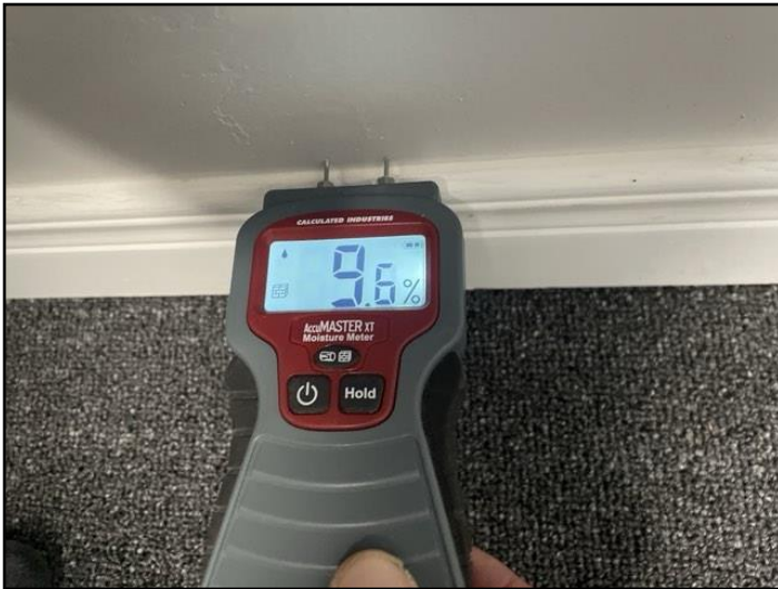
Rear - Typical reading noted - Dry
