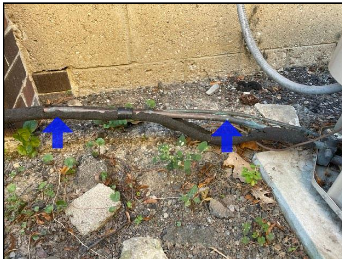
Insulation - missing
