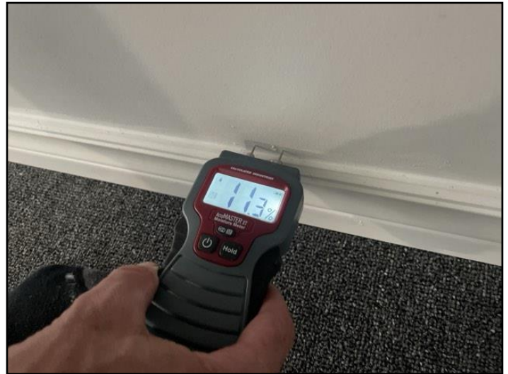
Right - Typical reading noted - Dry
