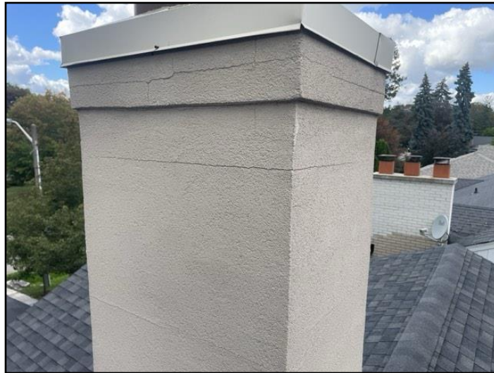
Minor cracks
