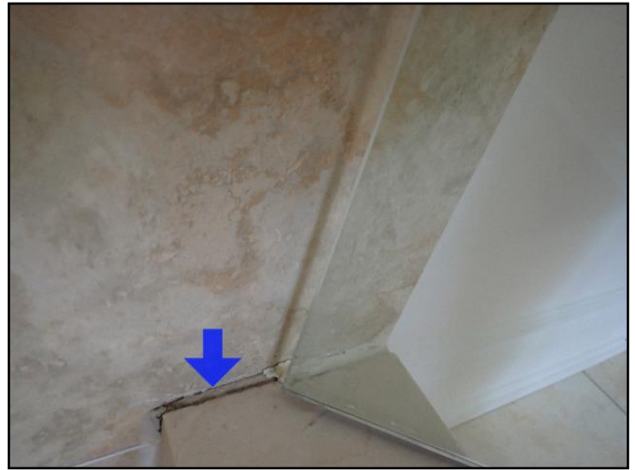
Second floor bathroom
